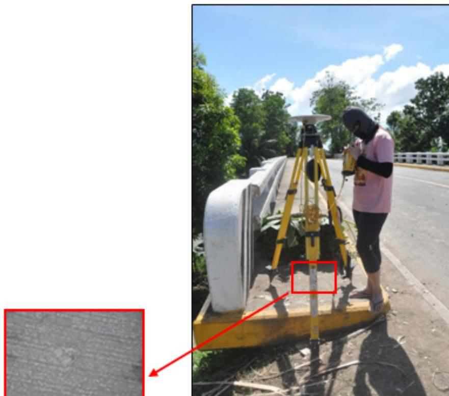
Figure 33. GNSS base receiver setup, Trimble® SPS 852, at NW-100 in Danao Bridge, Brgy. Jonobjonob, Escalante City, Negros Occidental
