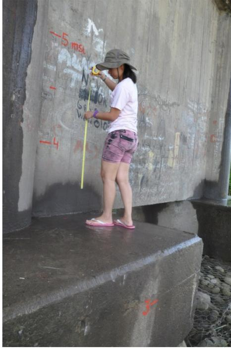
Figure 38. MSL markings on the Malogo Bridge pier
