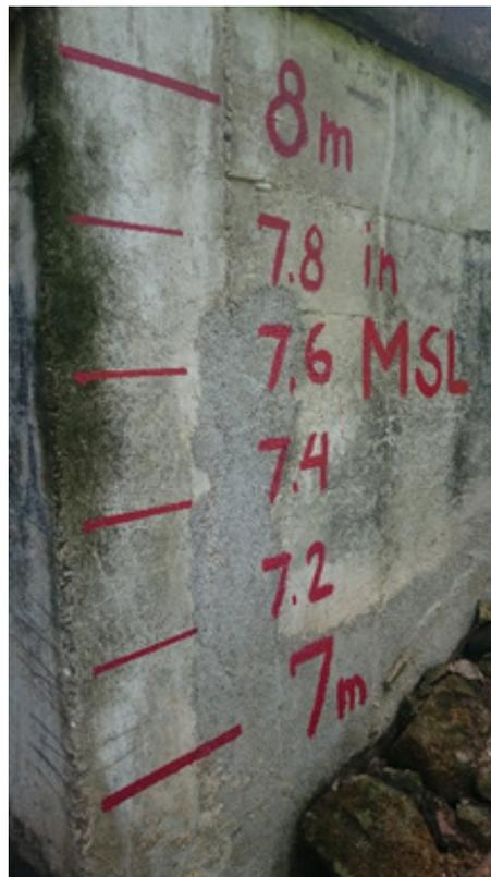
Figure 47. Water-level markings on Puente-Bunglas Bridge
