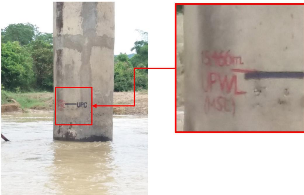
Figure 42. Water-level markings on Barasbarasan Bridge
