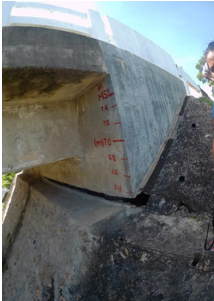
Figure 40. Water level markings on Tabuan Bridge.
