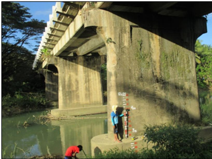
Figure 44. Water-level markings on Aborlan Bridge.
