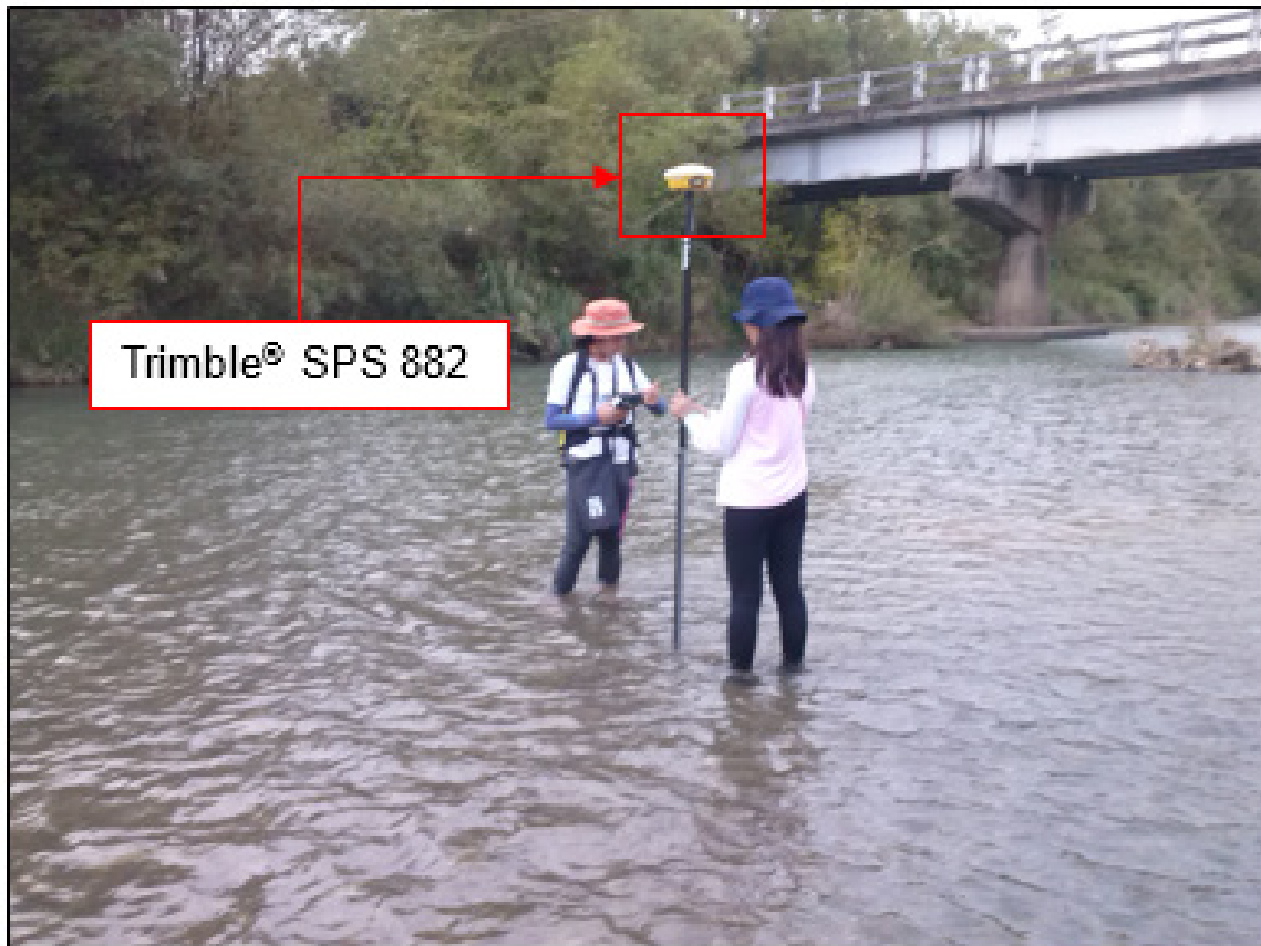
Figure 49. Gathering of random bathymetric points along Abra de Ilog River
