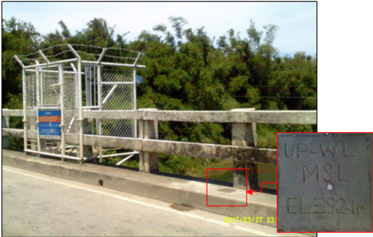
Figure 44. Water surface elevation marking on Lumang Bayan Bridge sidewalk
