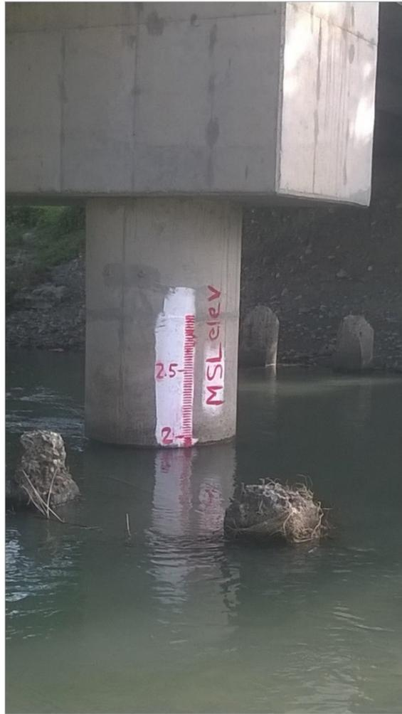
Figure 41. Water-level markings on the post of Baroc Bridge
