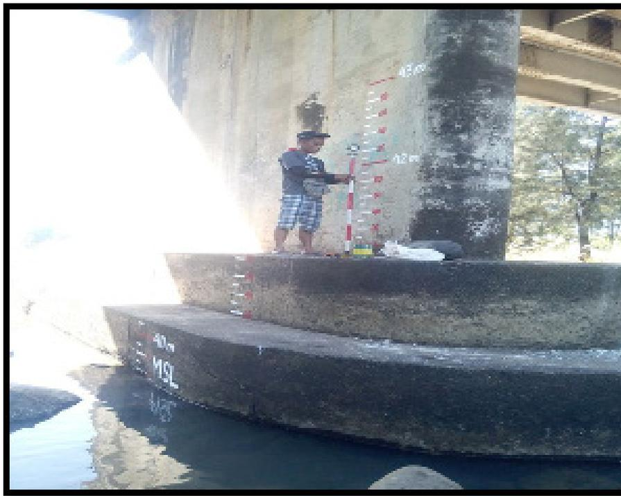
Figure 36. Water level markings on Batang-batang Bridge.
