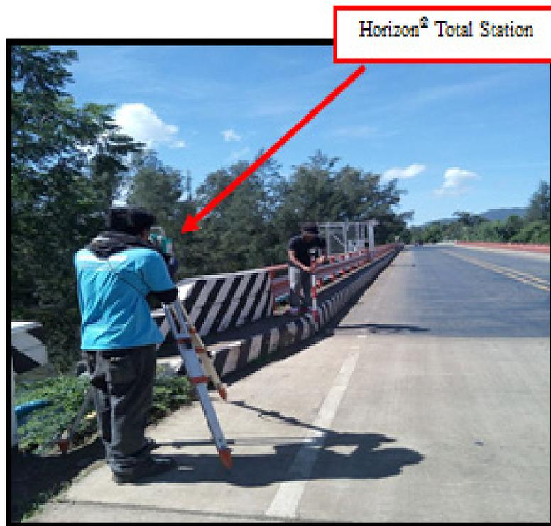
Figure 32. Bridge As-Built Survey of Batang-batang Bridge.
