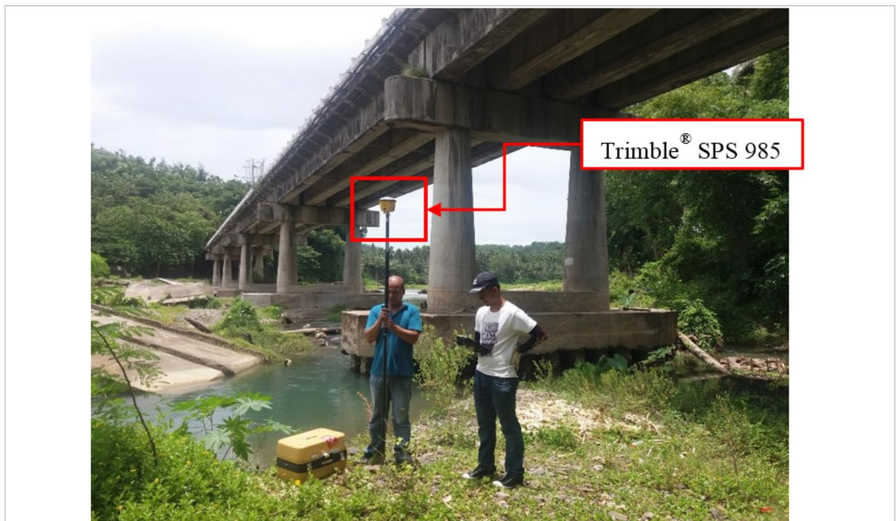
Figure 31. Bridge as-built survey, using PPK Technique
