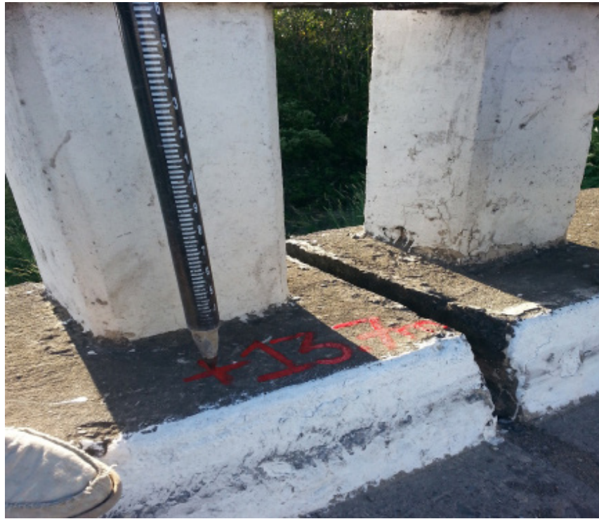
Figure 42. Water level marking at Caguray Bridge deck, Brgy. Poblacion, Municipality of Magsaysay
