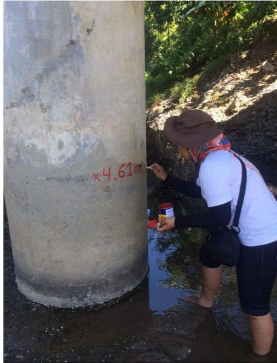
Figure 44. Water level marking at Alipid Bridge, Brgy. Sto. Niño, Municipality of Sablayan
