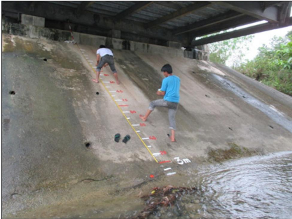
Figure 38. Water-level markings on Ilog-Ilog Bridge.
