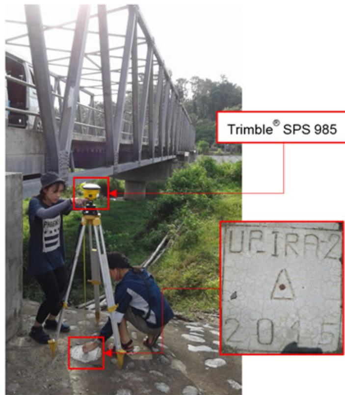
Figure 31. GNSS receiver set-up, Trimble® SPS 985, at UP\_IRA-2, located on the side of Iraan Bridge in Brgy. Iraan, Rizal, Province of Palawan.
