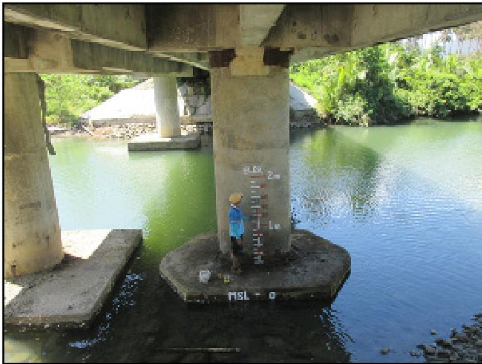
Figure 41. Water-level markings on Inagauan Bridge
