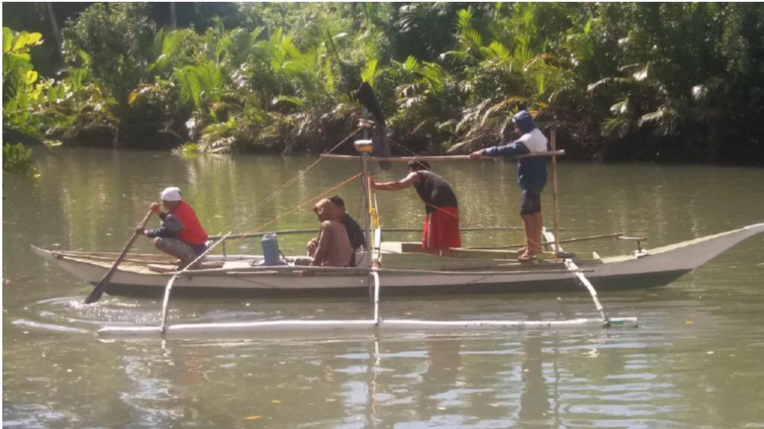
Figure 44. Manual Bathymetric survey using a Trimble® SPS 985 in GNSS PPK survey technique in Caramay River
