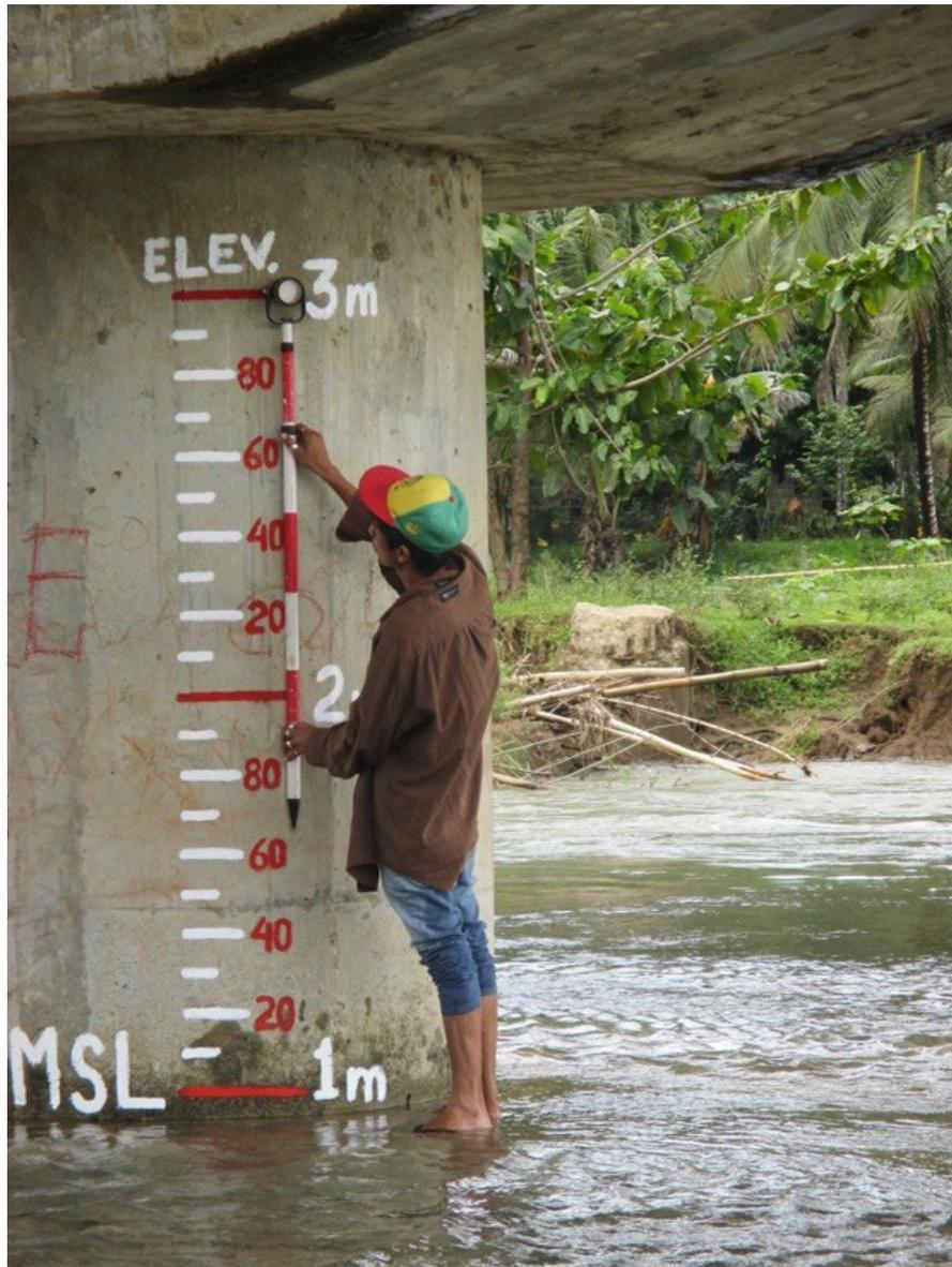
Figure 40. Water-level markings on Iraan Bridge
