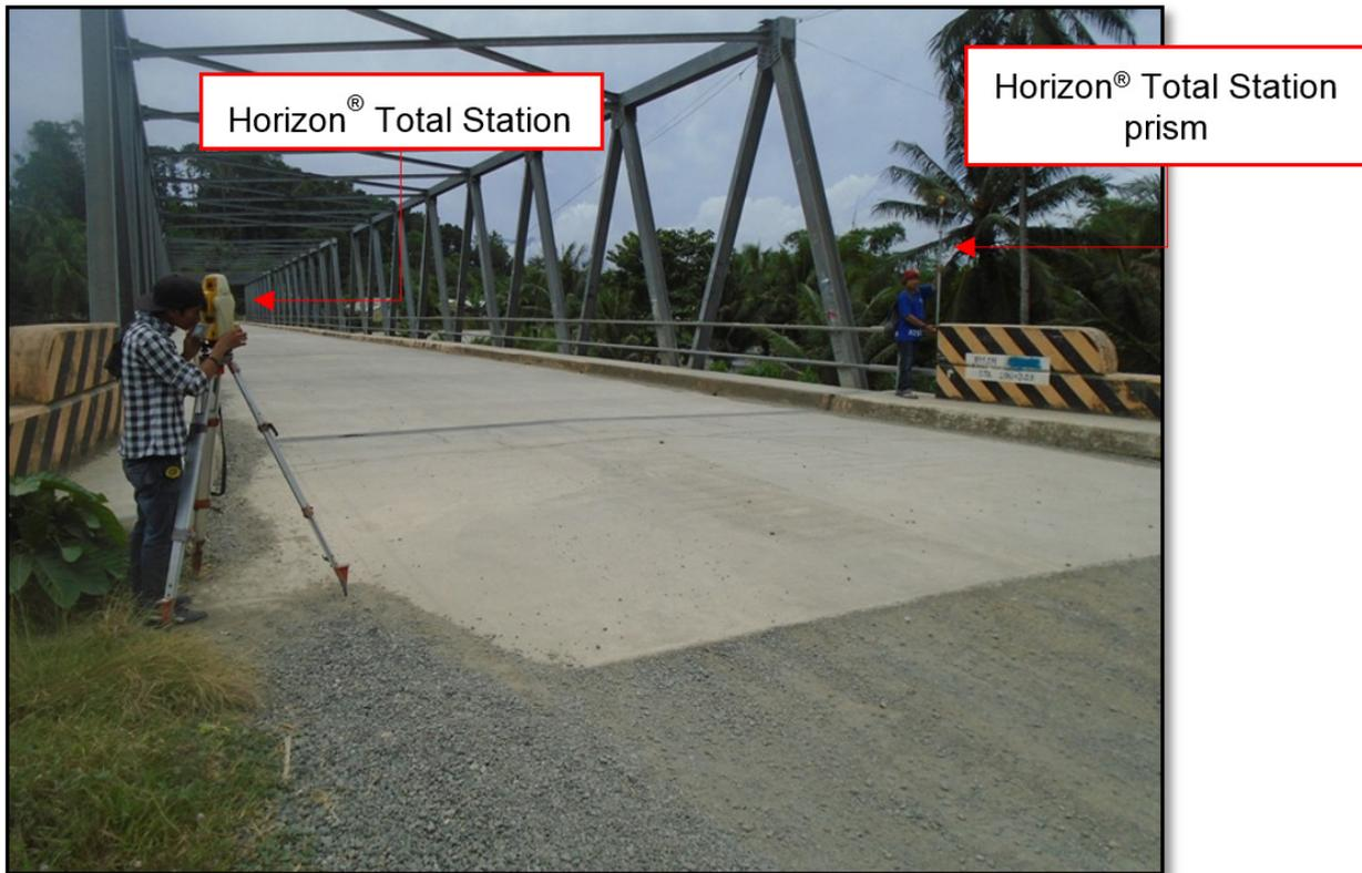
Figure 35. As-built survey of Iraan Bridge
