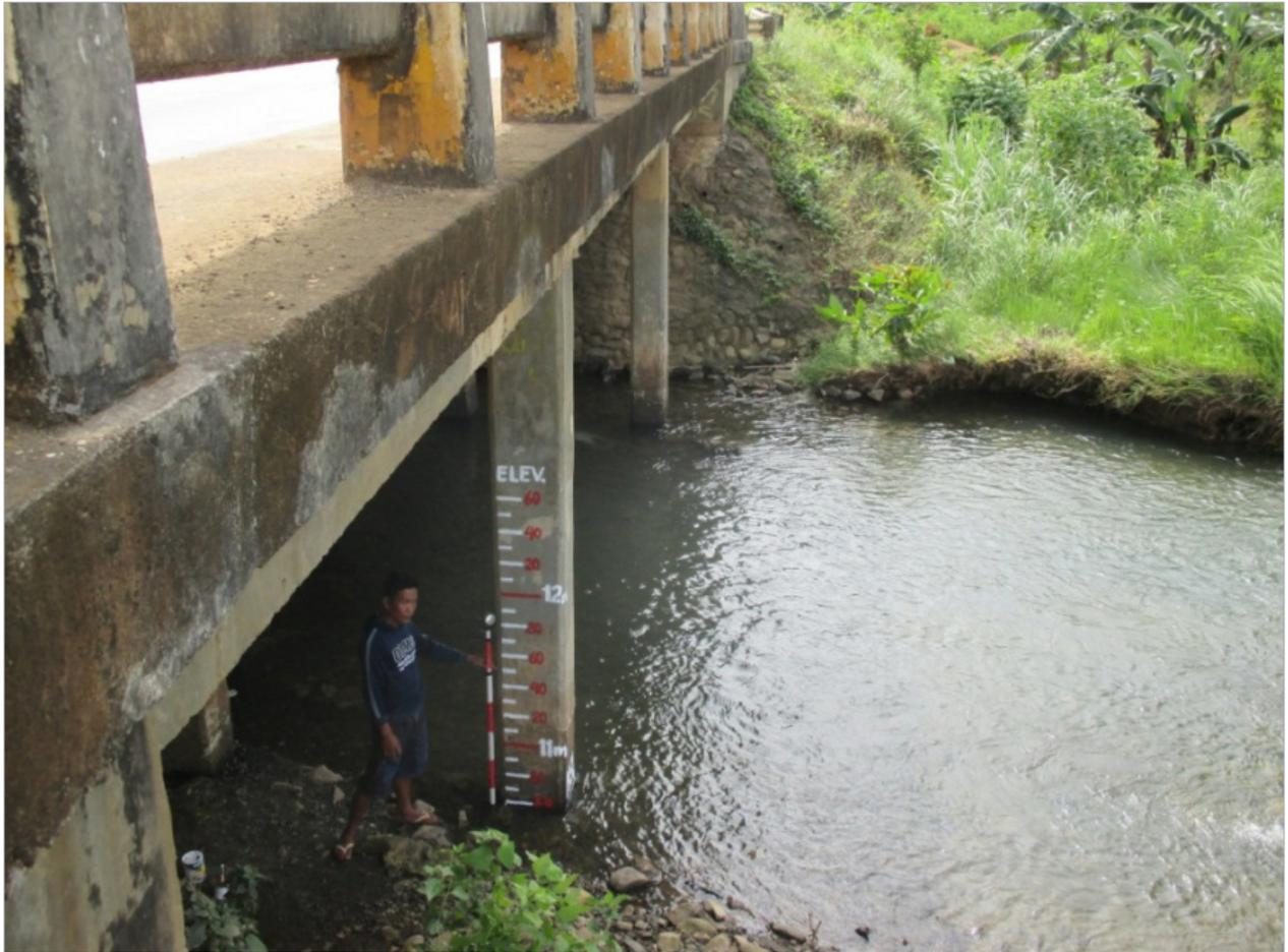
Figure 38. Water-level markings on Iwahig Brookes Bridge
