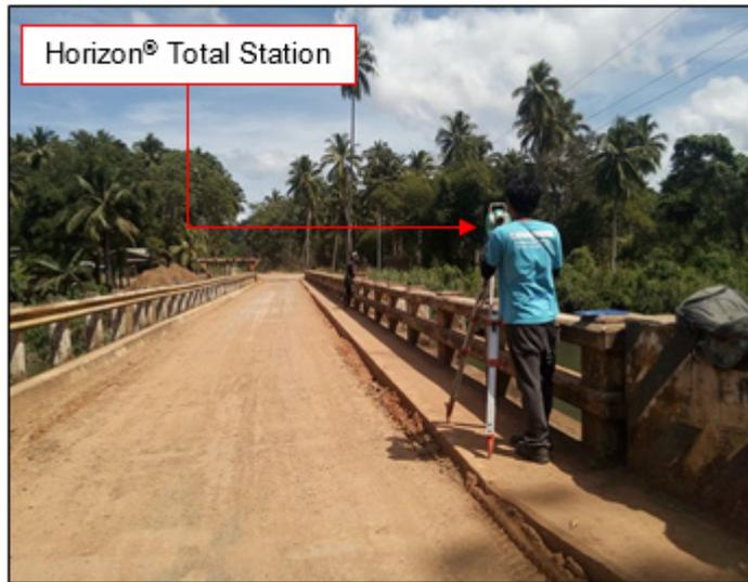
Figure 38. As-built survey of Iwahig Bridge
