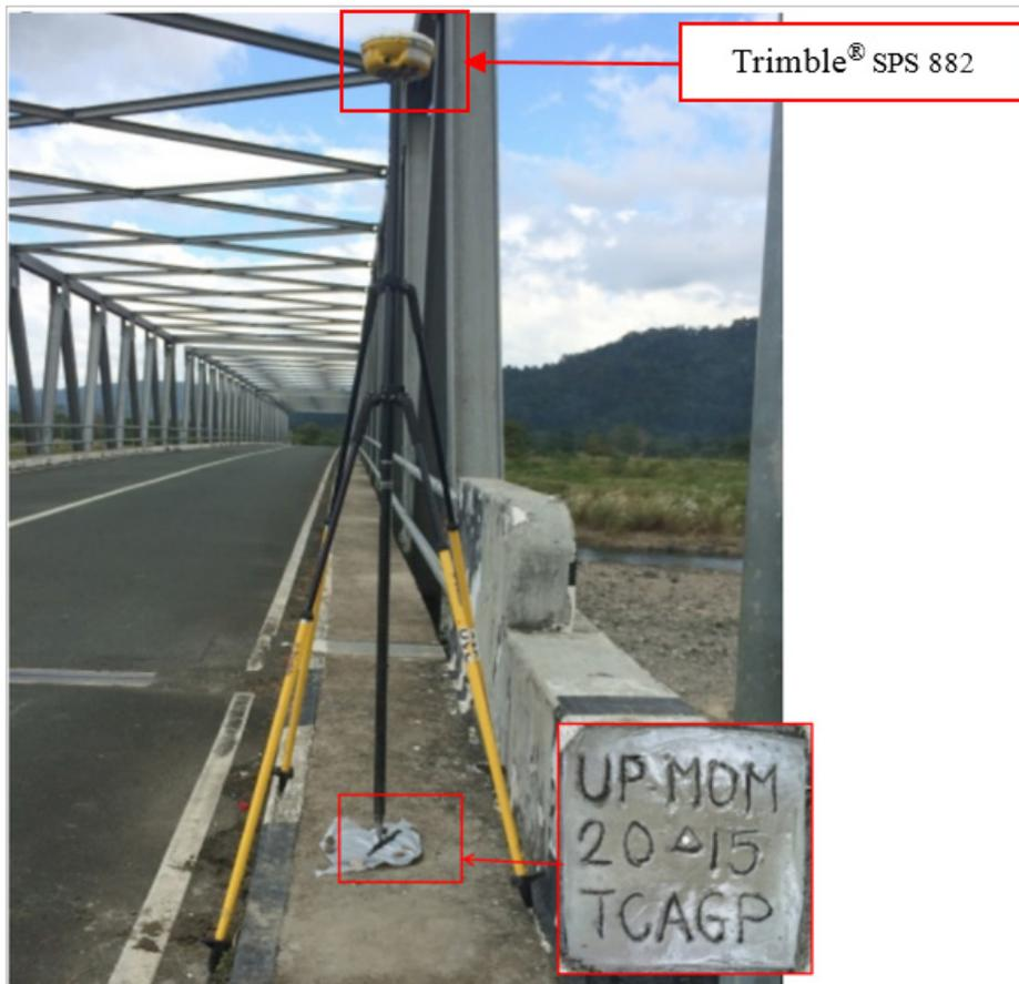
Figure 36. GNSS receiver set-up, Trimble® SPS 882, at UP-MOM, Mompong Bridge approached in Brgy. Lumang Bato, Municipality of Sablayan, Occidental Mindoro.
