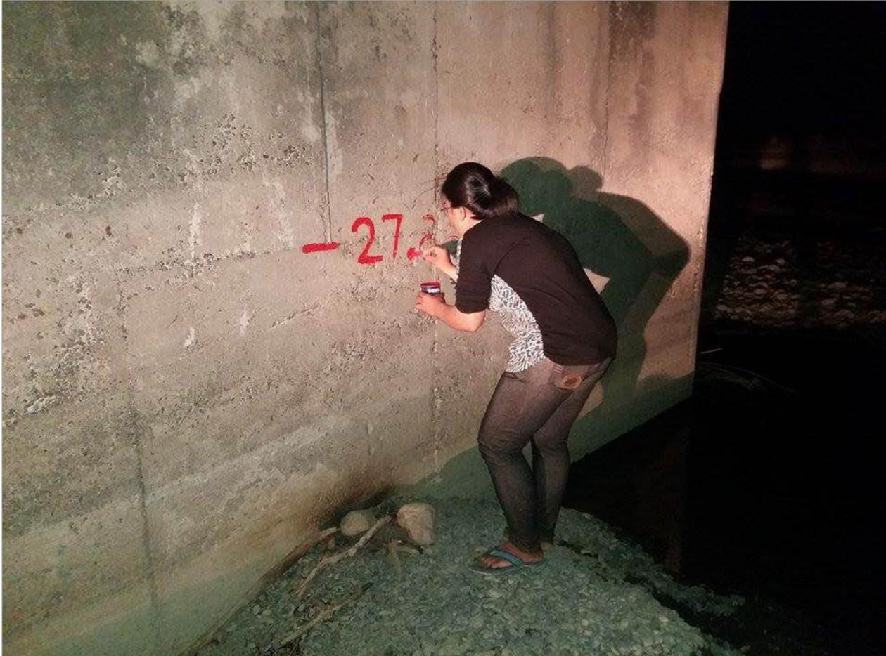
Figure 42. Water level marking at Lumintao Bridge's pier in Brgy. Magsikap, Municipality of Rizal
