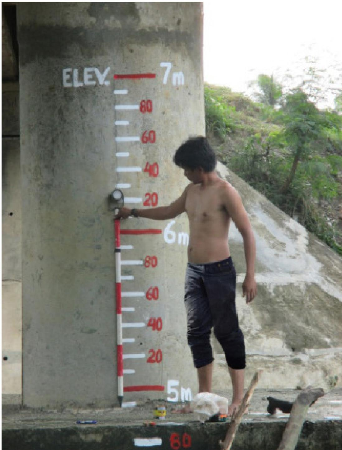
Figure 35. Water-level markings on Malambunga Bridge
