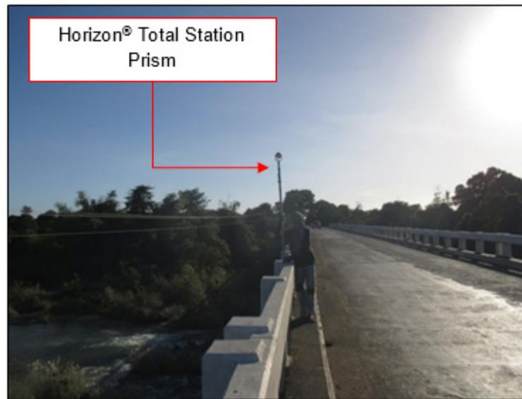
Figure 36. As-built survey of Malatgao Bridge
