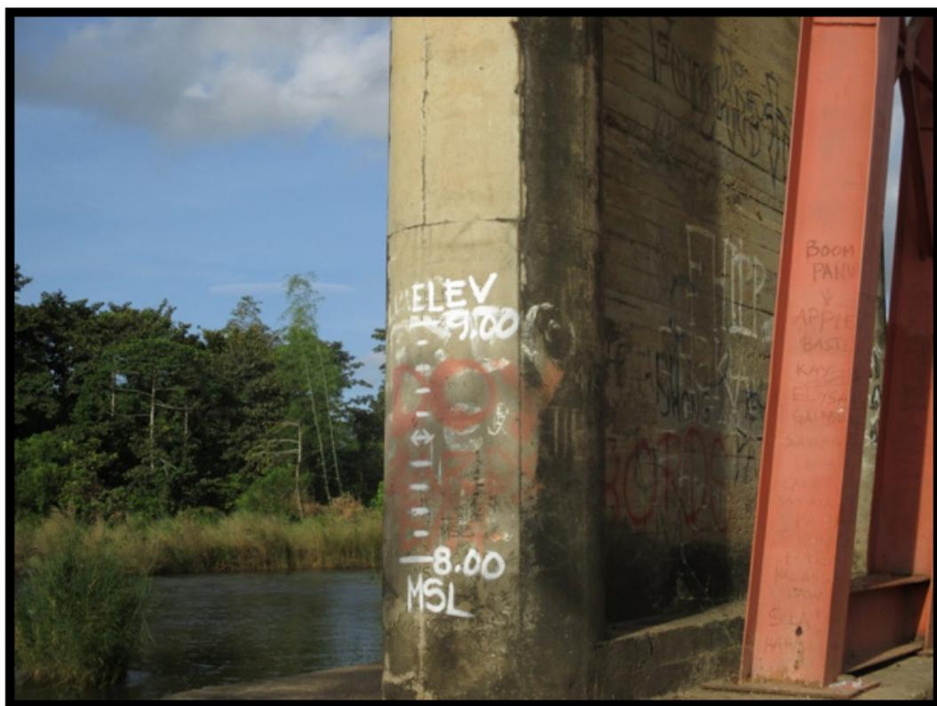
Figure 40. Water-level markings on Malatgao Bridge
