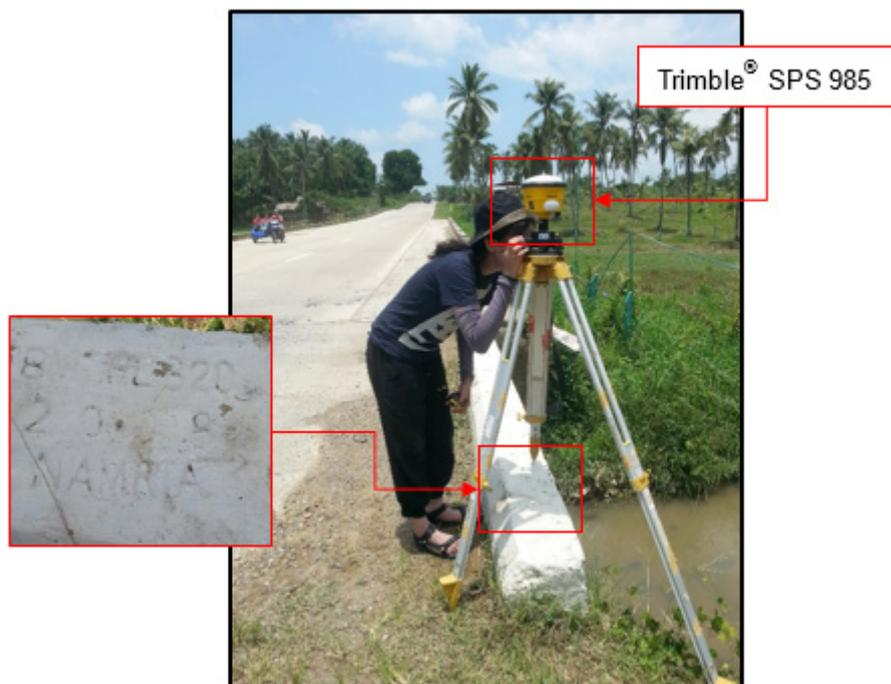
Figure 29. GNSS receiver set up, Trimble® SPS 985, at PL-320, located on top of a culvert headwall along the National Road in Brgy. Ramon Magsaysay, Aborlan, Province of Palawan
