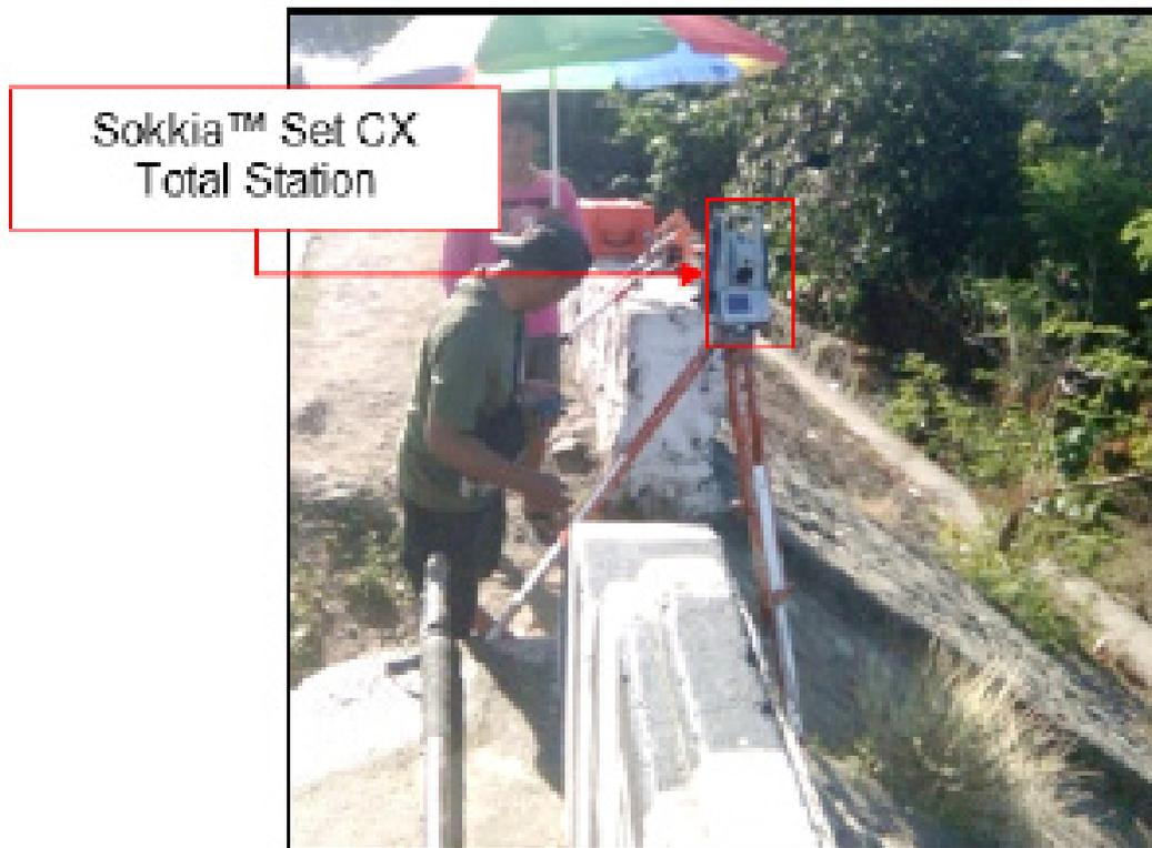
Figure 39. Cross-section survey of Mamburao Bridge
