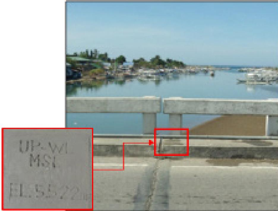
Figure 43. Water surface elevation marking on Mamburao Bridge sidewalk
