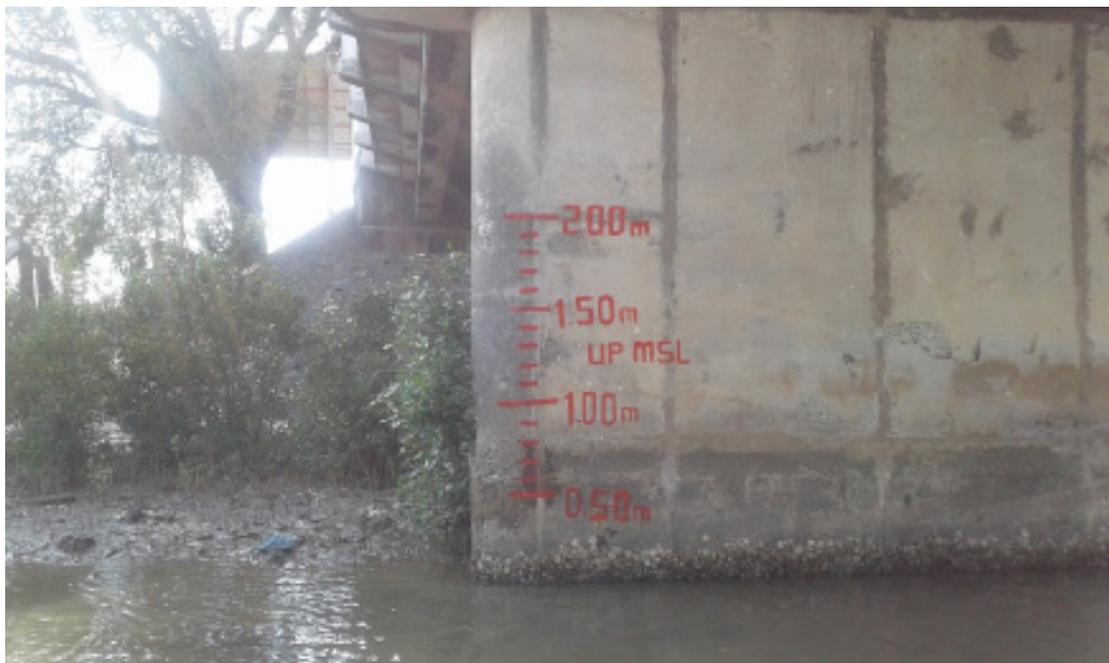
Figure 44. Water level markings on the pier of Mamburao Bridge
