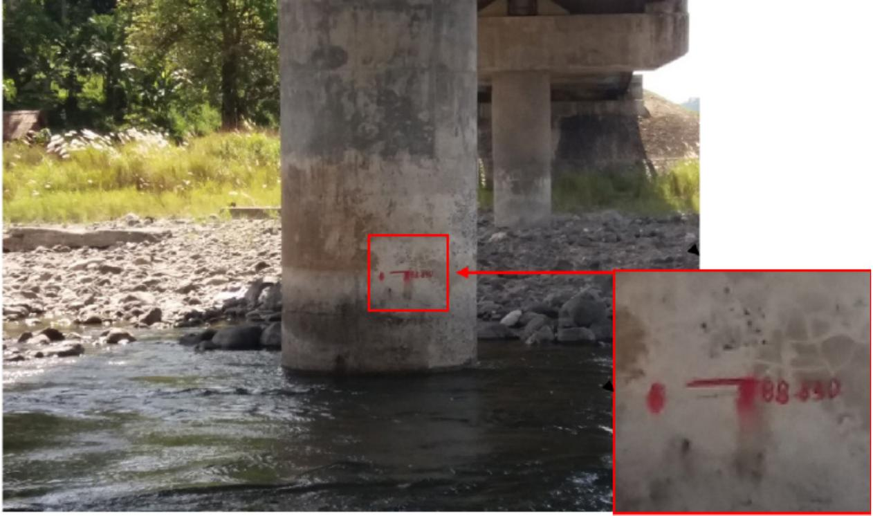
Figure 44. Water-level marking at Mompong Bridge, Brgy. Sta. Lucia, Municipality of Sablayan
