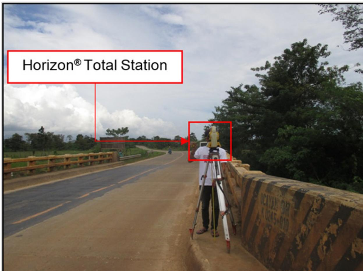
Figure 36. As-built survey of Ocayan Bridge.
