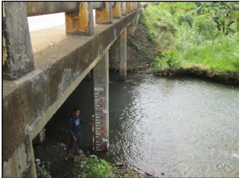
Figure 40. Water-level markings on Ocayan Bridge.
