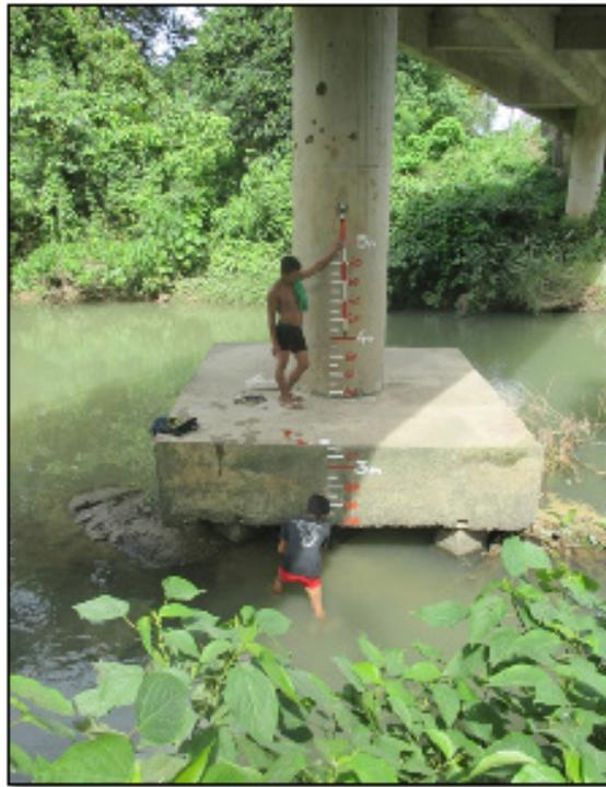
Figure 38. Water-level markings on Panitian Bridge
