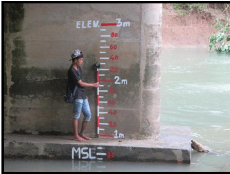
Figure 36. Water-level markings on Pulot Bridge
