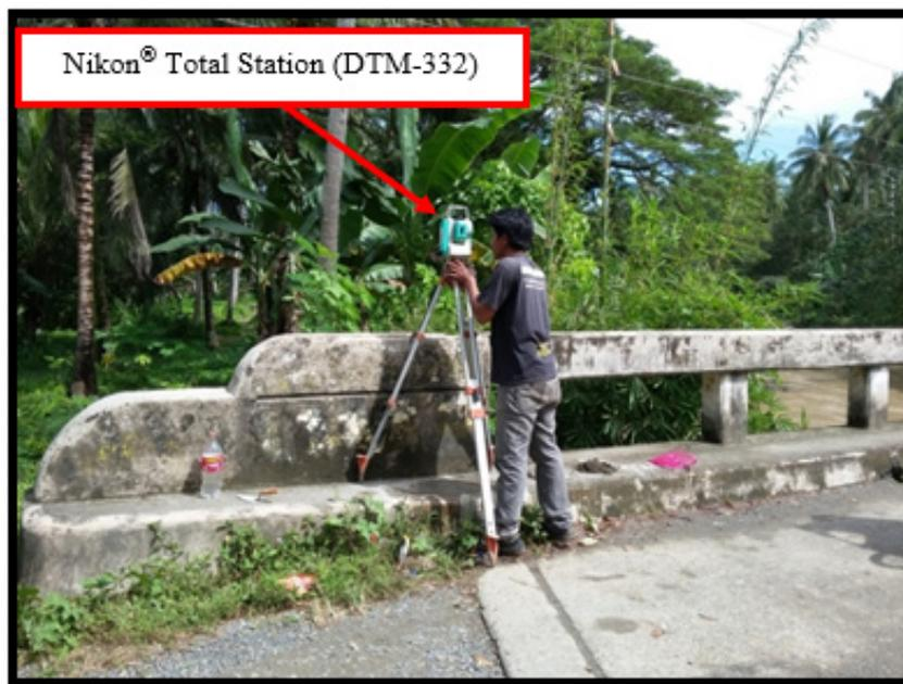
Figure 32. As-built survey of Pulot Bridge
