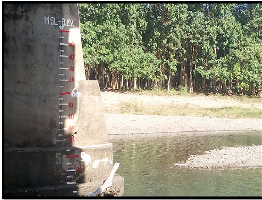
Figure 38. Water-level markings on Tigaplan Bridge
