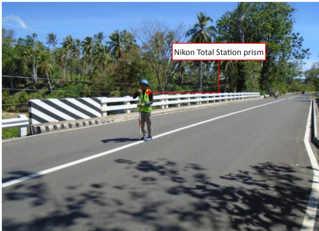
Figure 36. As-built survey of Bitanagan Bridge
