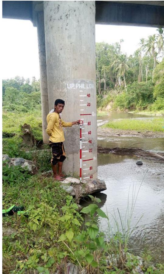
Figure 41. Water-level markings on Bitanagan Bridge
