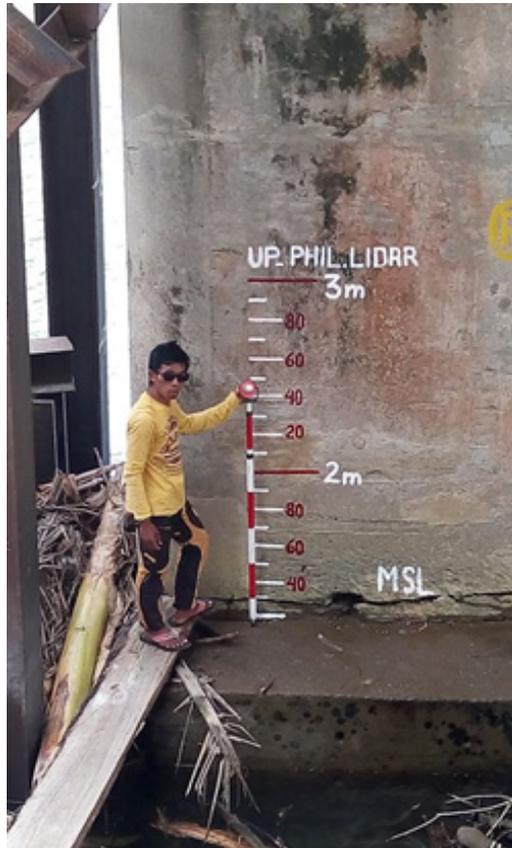
Figure 40. Water-level markings on Caraga Bridge
