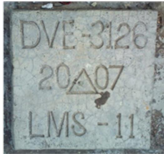
Figure 2. GPS set-up over DVE-3126 located inside the compound of Kinablangan Barangay Hall (a) and NAMRIA reference point DVE-3126 (b) as recovered by the field team.
