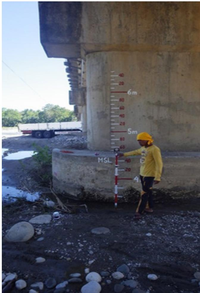
Figure 40. Water-level markings on Casauaman Bridge.
