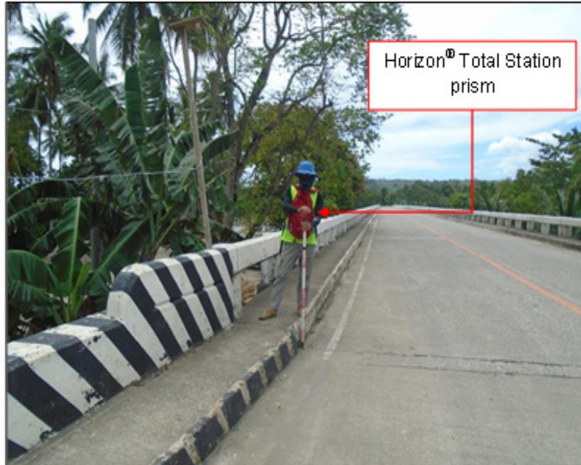
Figure 35. As-built survey conducted at Casauman Bridge.
