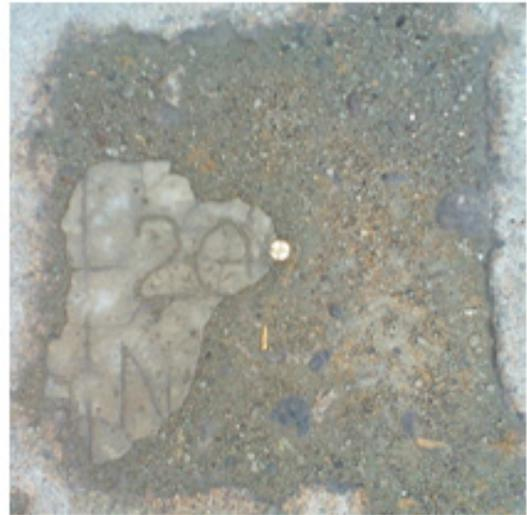
Figure 7. GPS set-up over NW-123 in Cadiz, Negros Occidental going to San Carlos, along the national road (a) and NAMRIA reference point NW-123 (b) as recovered by the field team.
