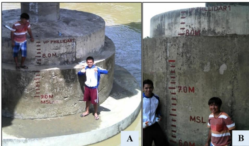
Figure 42. Water level mark at the left (A) and right (B) piers of the Lasang Bridge, facing downstream
