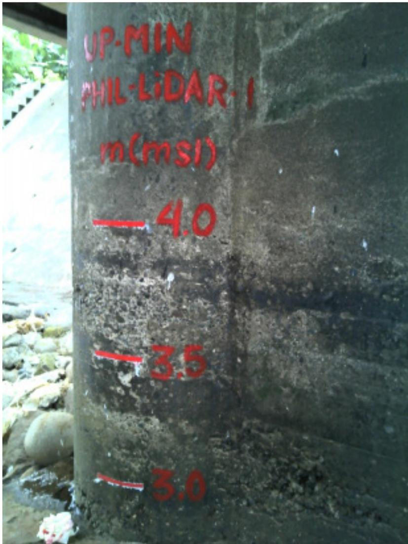
Figure 43. Water level markings on the post of Lipadas Bridge II
