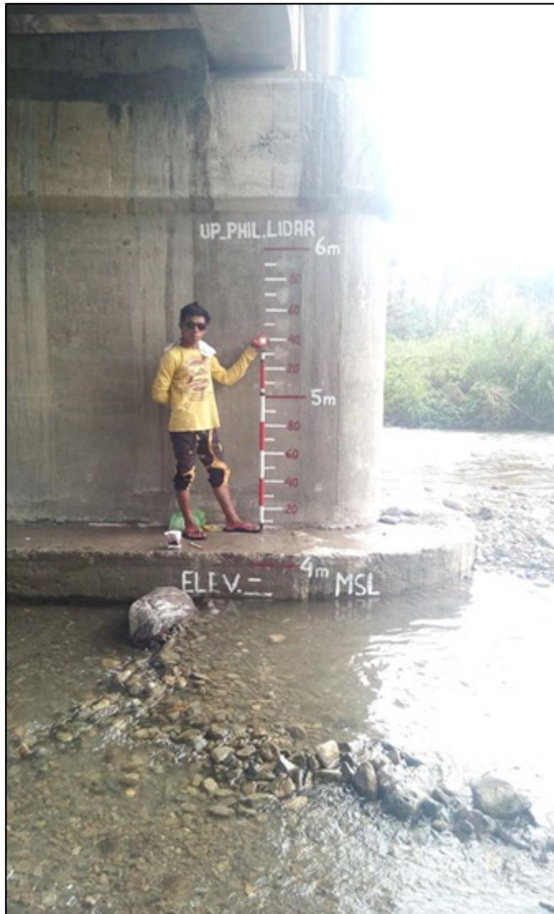
Figure 40. Water level markings on Mayo Bridge
