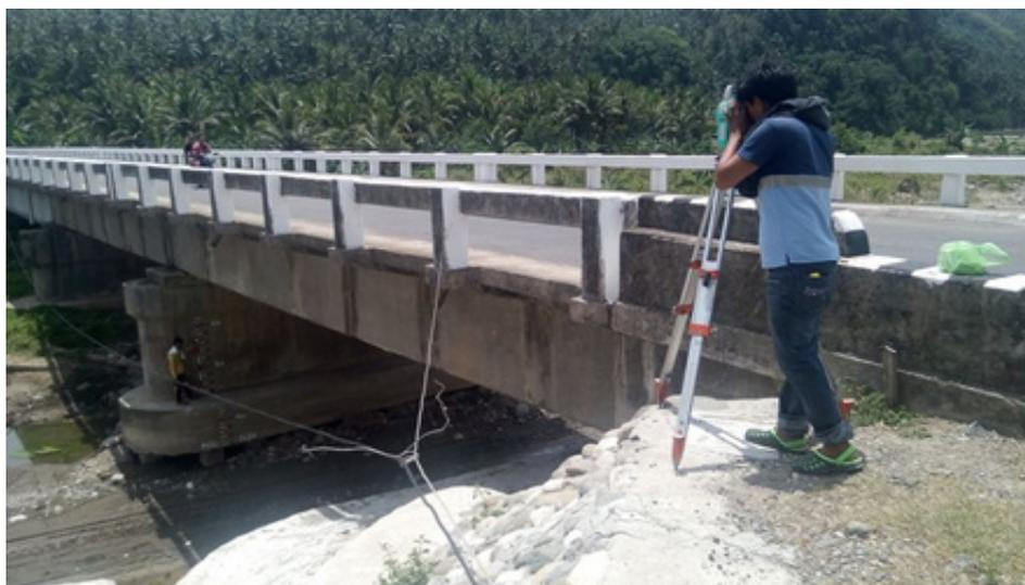
Figure 36. As-built survey of Quinonoan Bridge.
