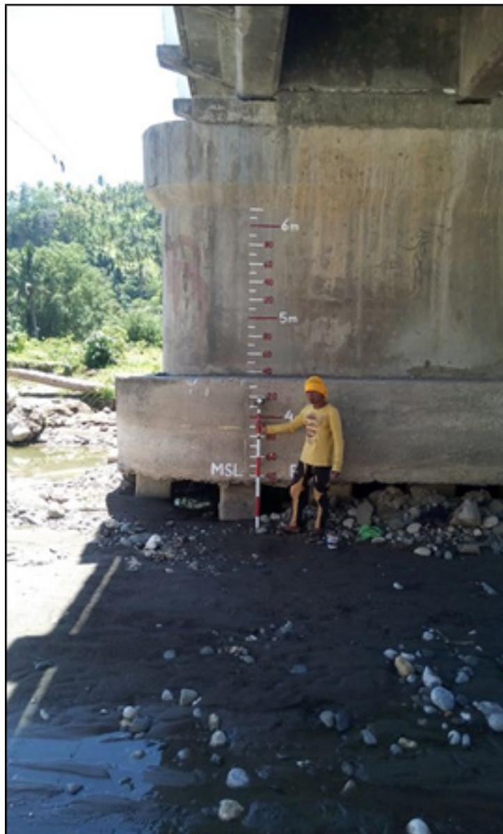
Figure 40. Water-level markings on Quinonoan Bridge.
