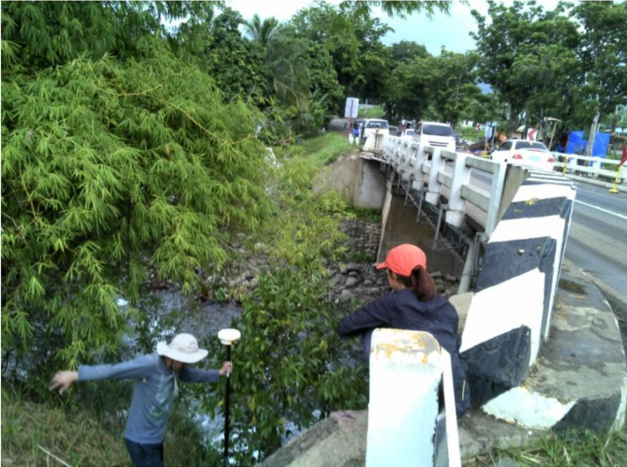
Figure 38. Cross-section and bridge as-built survey at the downstream side of Cebulan Bridge, Brgy. Astorga, Santa Cruz, Davao del Sur
