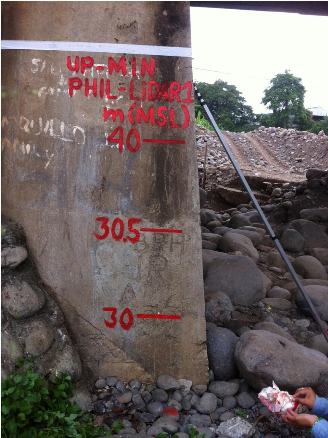
Figure 42. Water level markings on Cebulan Bridge
