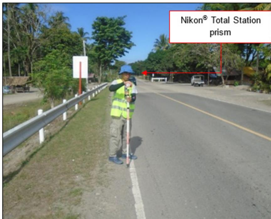
Figure 34. The cross-section survey conducted at the Sumlog Bridge.
