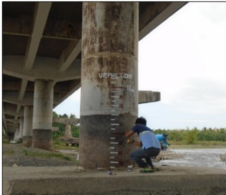
Figure 38. Painting of water level markings on Sumlog Bridge.
