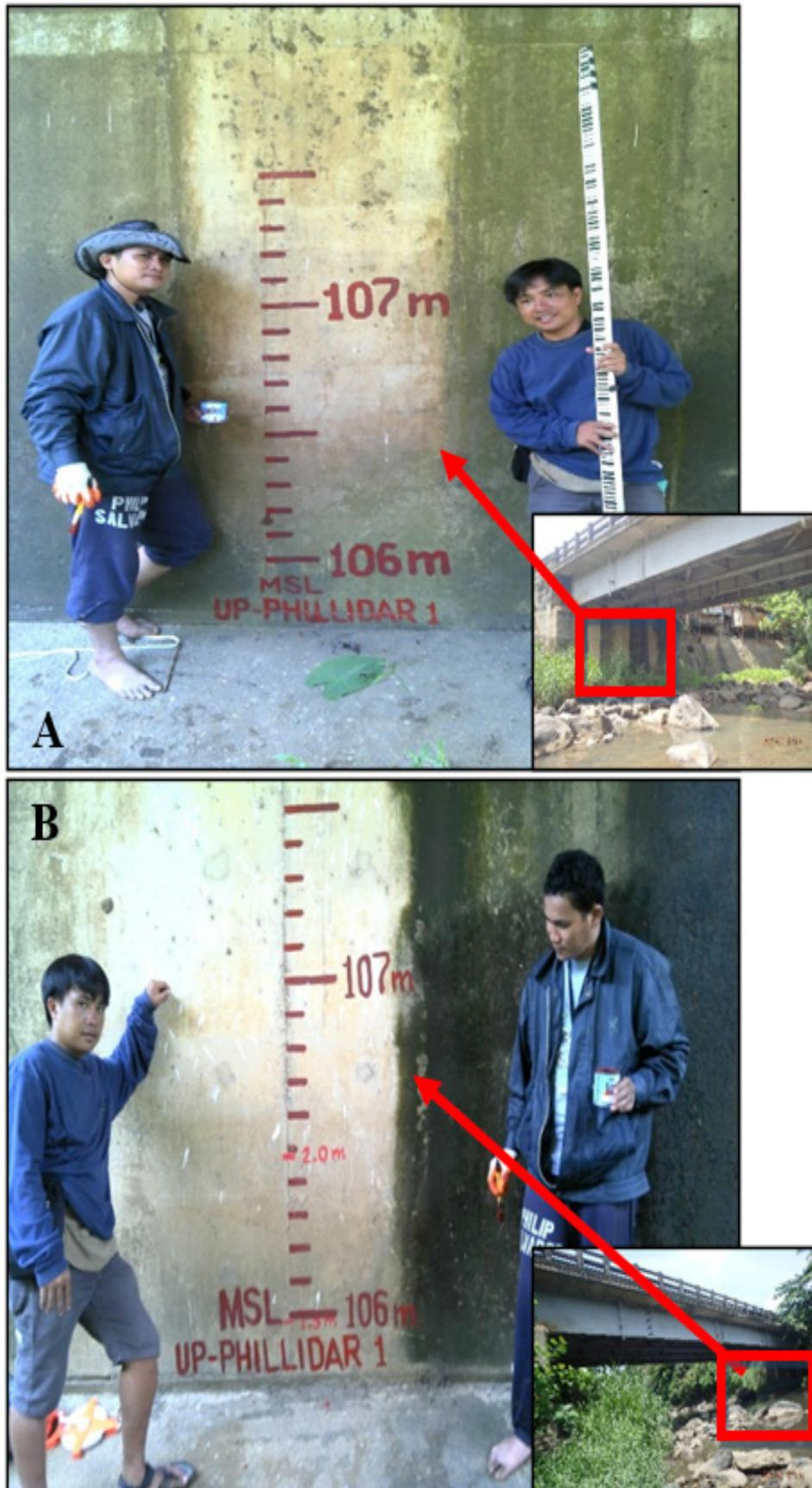
Figure 45. Water Level marking at the left (A) and right pier (B) of the bridge facing downstream of Mintal Bridge
