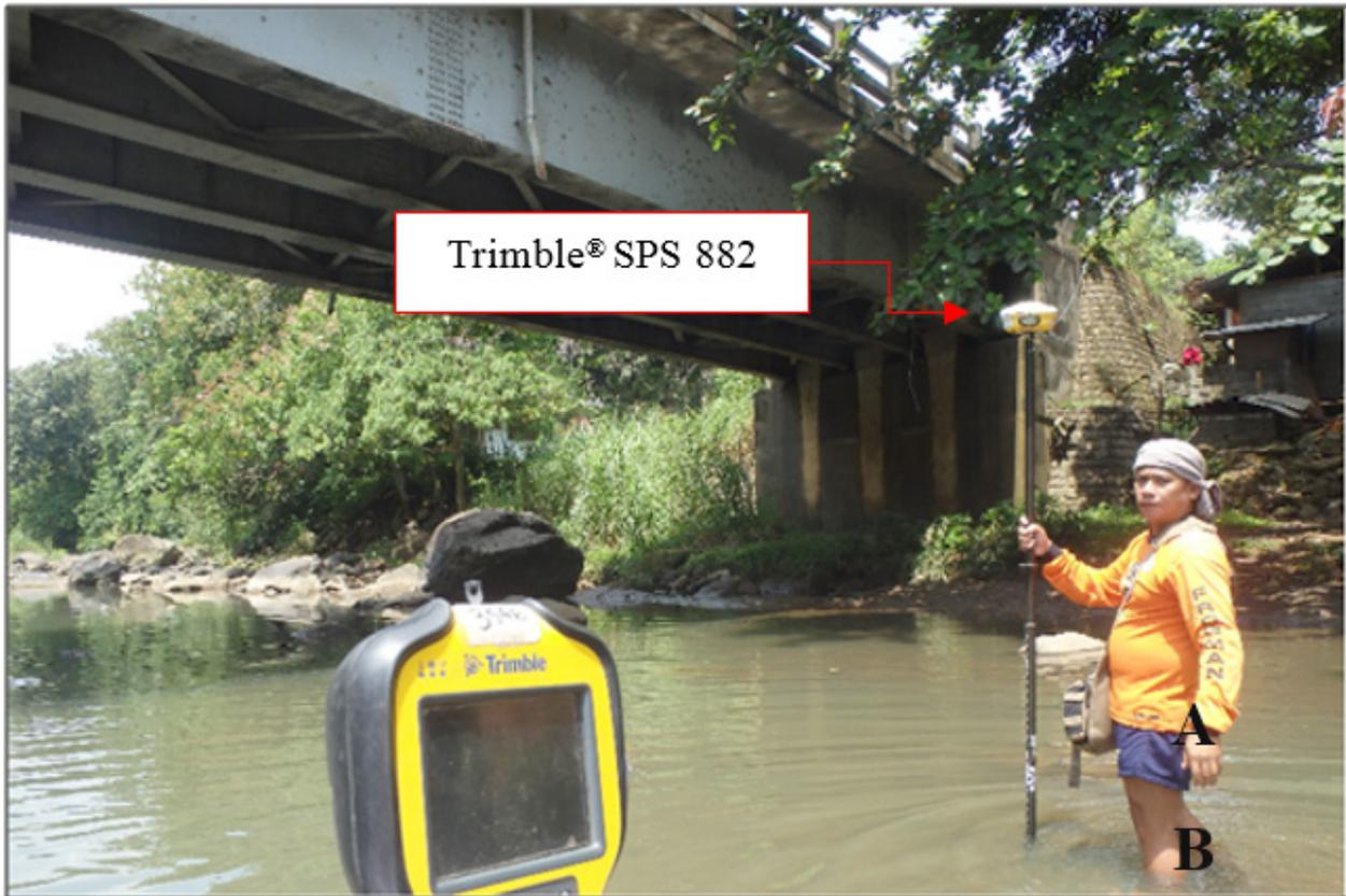
Figure 37. Cross-section Survey at Mintal Bridge
