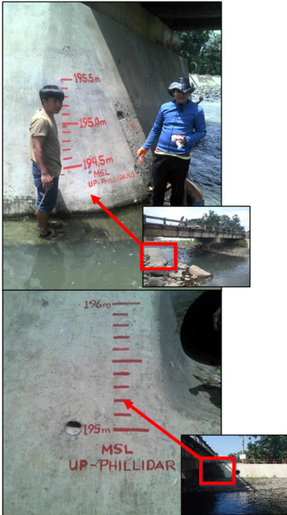
Figure 44. Water level markings on Talomo Bridge
