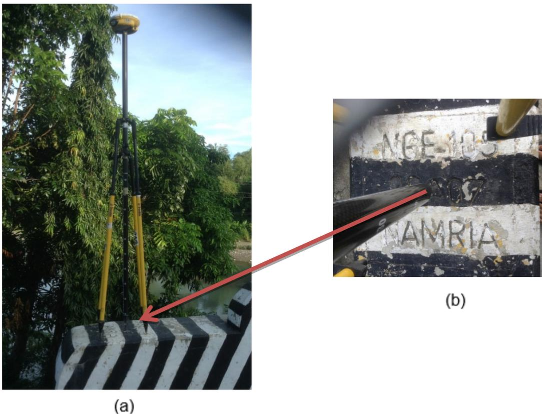
Figure 7 GPS set-up over NE-90 on a concrete sidewalk of Guinsuan Bridge, 4 meters from the road centerline in Barangay Poblacion under the Municipality of Zamboanguita (a) and NAMRIA benchmark NE-90 (b) as recovered by the field team
