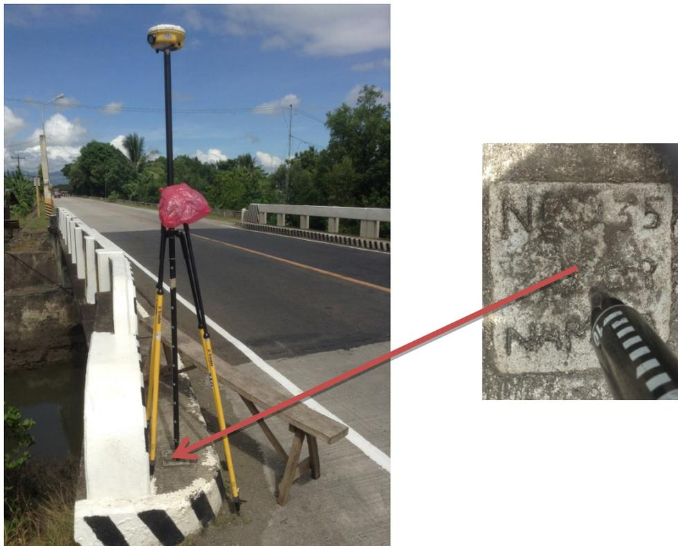
Figure 9 GPS set-up over NE-135 in Busuang Bridge on top of concrete sidewalk in Barangay Bio-os under the Municipality of Amlan (a) and NAMRIA benchmark NE-135 (b) as recovered by the field team.
