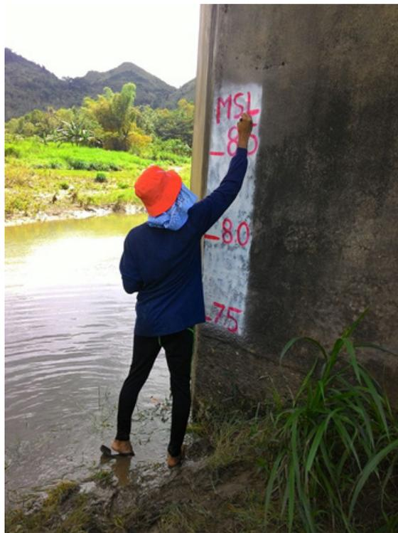
Figure 45. Water level marking on Guinabasan Bridge
