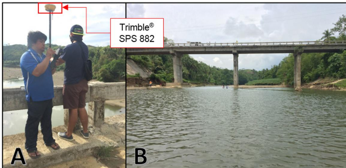
Figure 33. Cross-section and bridge as-built survey (a) for Baguhan Bridge, Brgy. Inabanga, Balilihan Bohol; Panoramic view (b) of the Baguhan Bridge.
