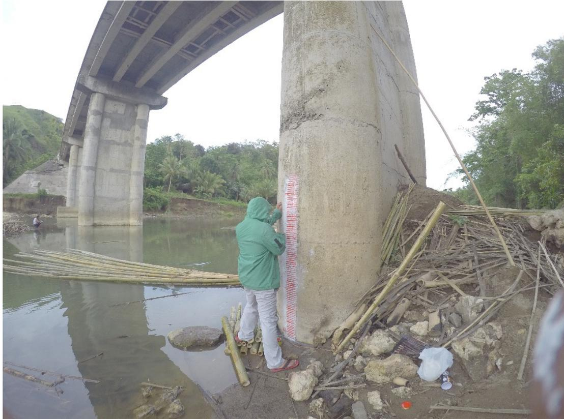
Figure 37. Water-level markings on the post of Baguhan Bridge.
