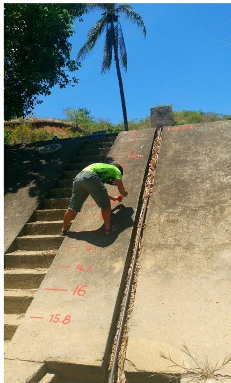
Figure 36. Water-level marking on Tiabanan River
