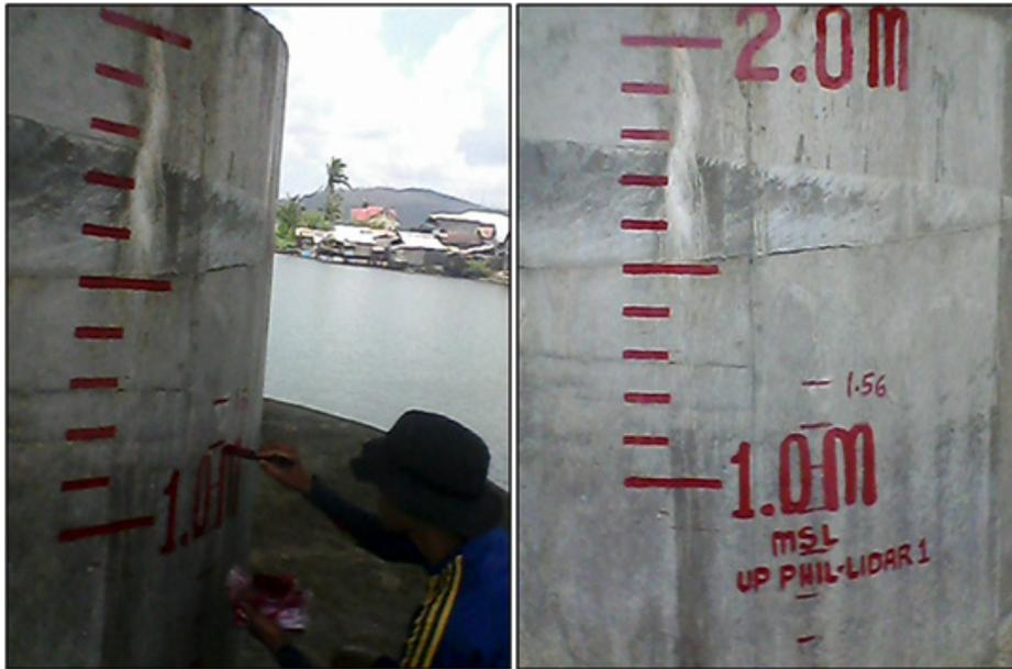
Figure 47. (A) Actual and (B) finished MSL water level markings on the Balangiga Bridge's pier
