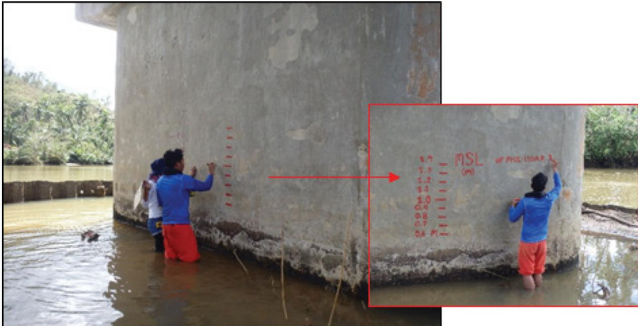
Figure 48. Finished Water Level Markings at Basey Bridge, Brgy. Guirang, Basey, Samar
