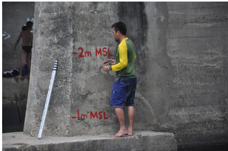
Figure 41. Water level marking of Daguitan Bridge's Pier
