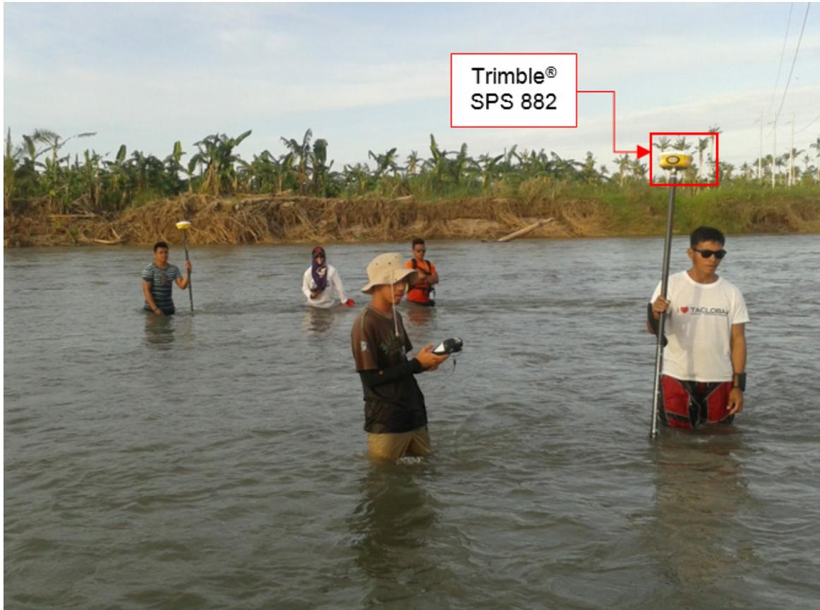
Figure 47. Manual bathymetric survey of Daguitan River
