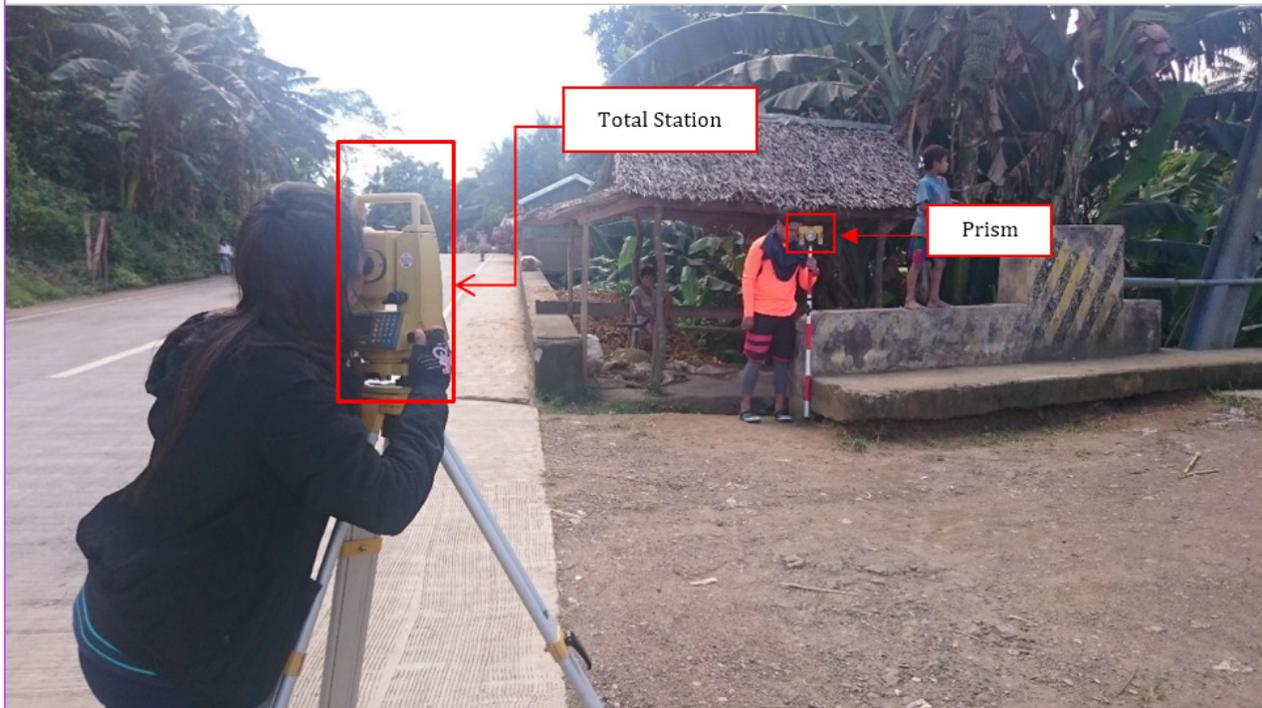
Figure 31. Bridge as-built and cross-section survey on the downstream side of the Cagbayang Bridge in Barangay Cagbayang, Oquendo District, Calbayog City
