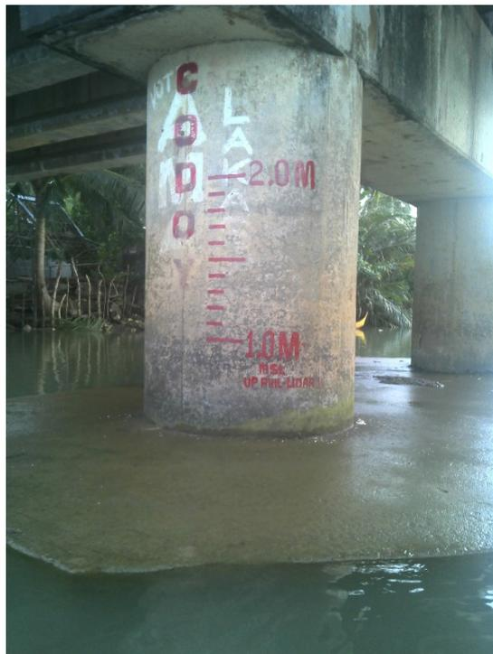
**Figure 43.** Actual (A) and finished (B) MSL water level markings in Llorente Bridge's Pier
