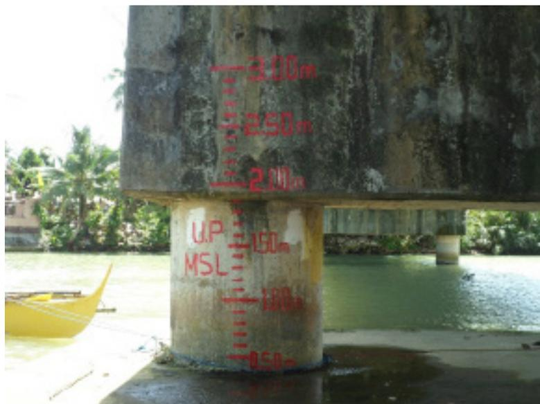
Figure 47. Water level markings on the pier of Loom Bridge
