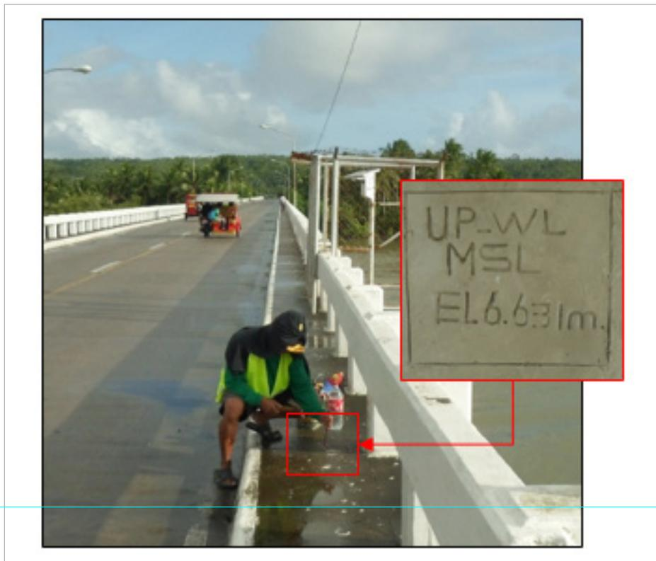
Figure 37. Water surface elevation marking on Oras Bridge sidewalk
