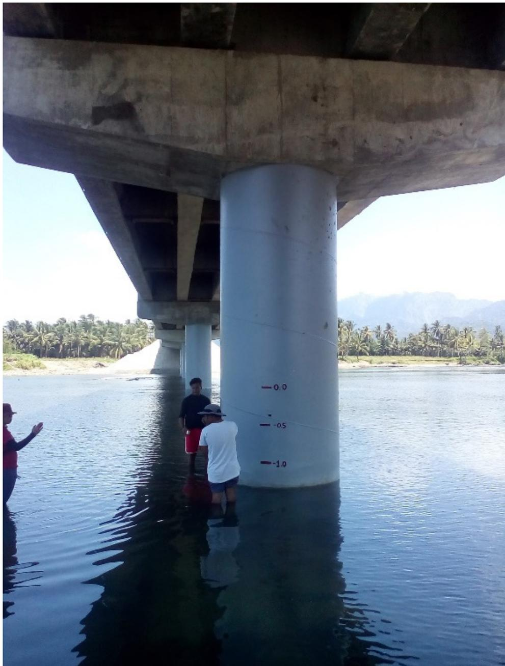
Figure 36. Water level marking at Pagbanganan Bridge
