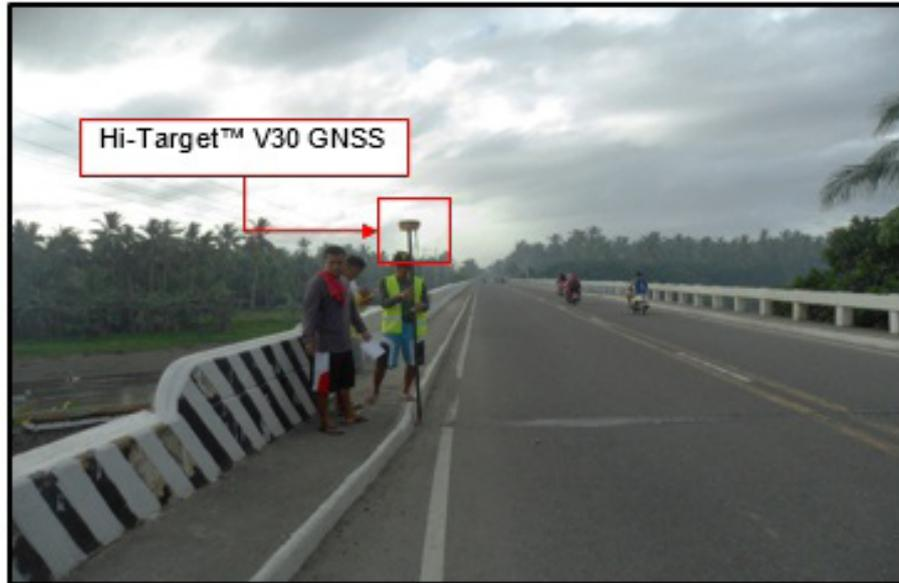
Figure 36. As-built survey of Salug Bridge
