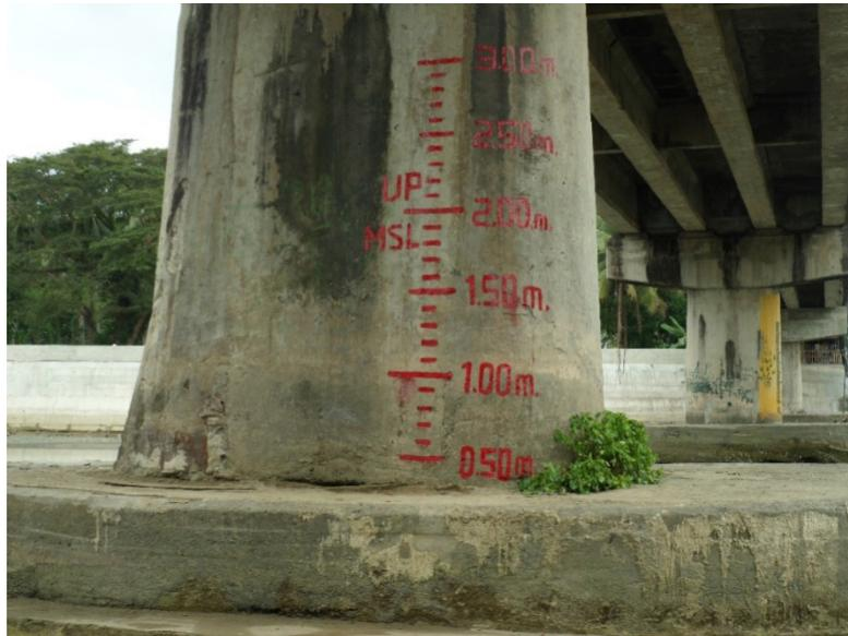
Figure 40. Water level marking at Salug Bridge
