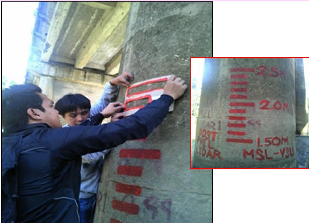
Figure 48. Painting of water level markings on Silaga Bridge
